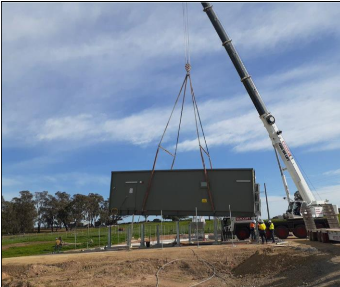
Delivery of the Solar Farm Substation High Voltage Switch Room
