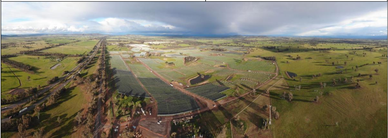
Aerial photo of current construction works
