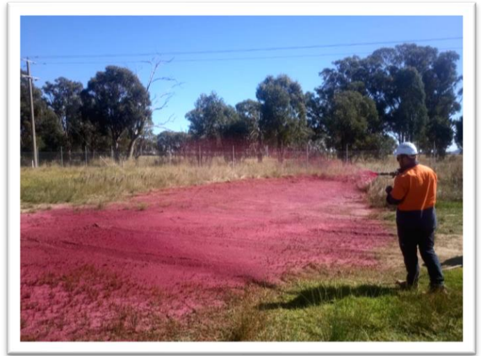
Spray on hydro mulch is applied to batters around the substation to restore grass cover.
