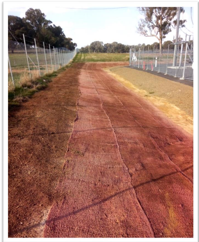
Spray on hydro mulch is applied to batters around the substation to restore grass cover.
