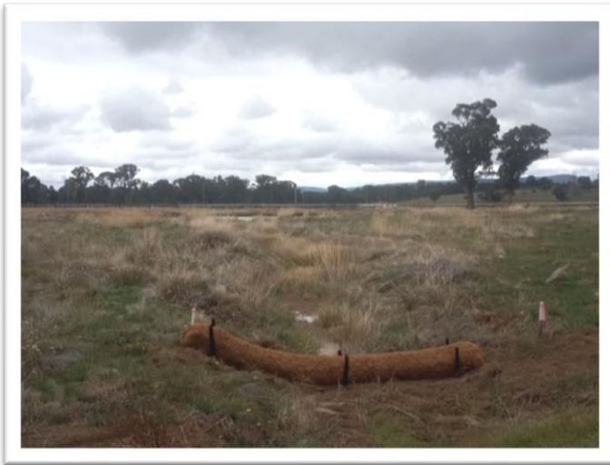
Natural coir logs have been sourced to prevent erosion onsite.
