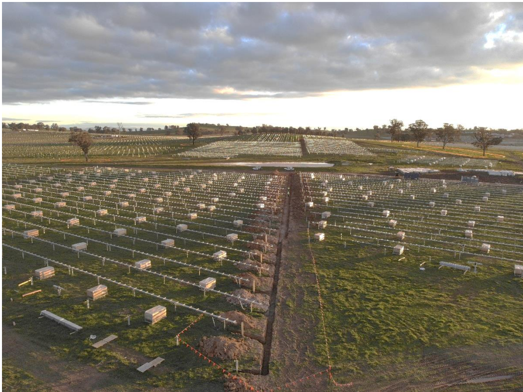
Winton Solar Farm construction site
