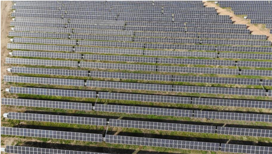
Block 2 solar array – all panels now rotate in sync with the sun.
