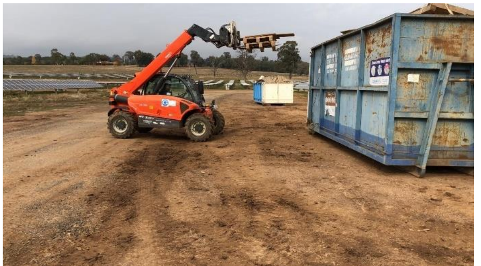
The last bins of timber pallets are sent offsite for recycling.
