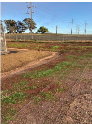
Seeded grass on sloped areas around the substation is starting to emerge.
