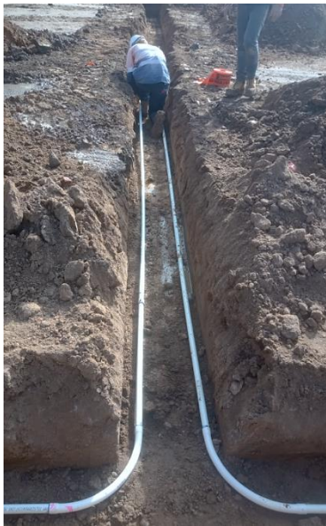
Communications cabling installation.
