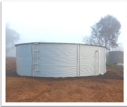
Our new water storage tank, recently installed by Hunkin Water Cartage.
